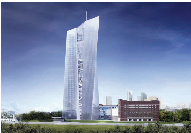
View of the new ECB premises from the east. Building work is due to be completed in 2014.
